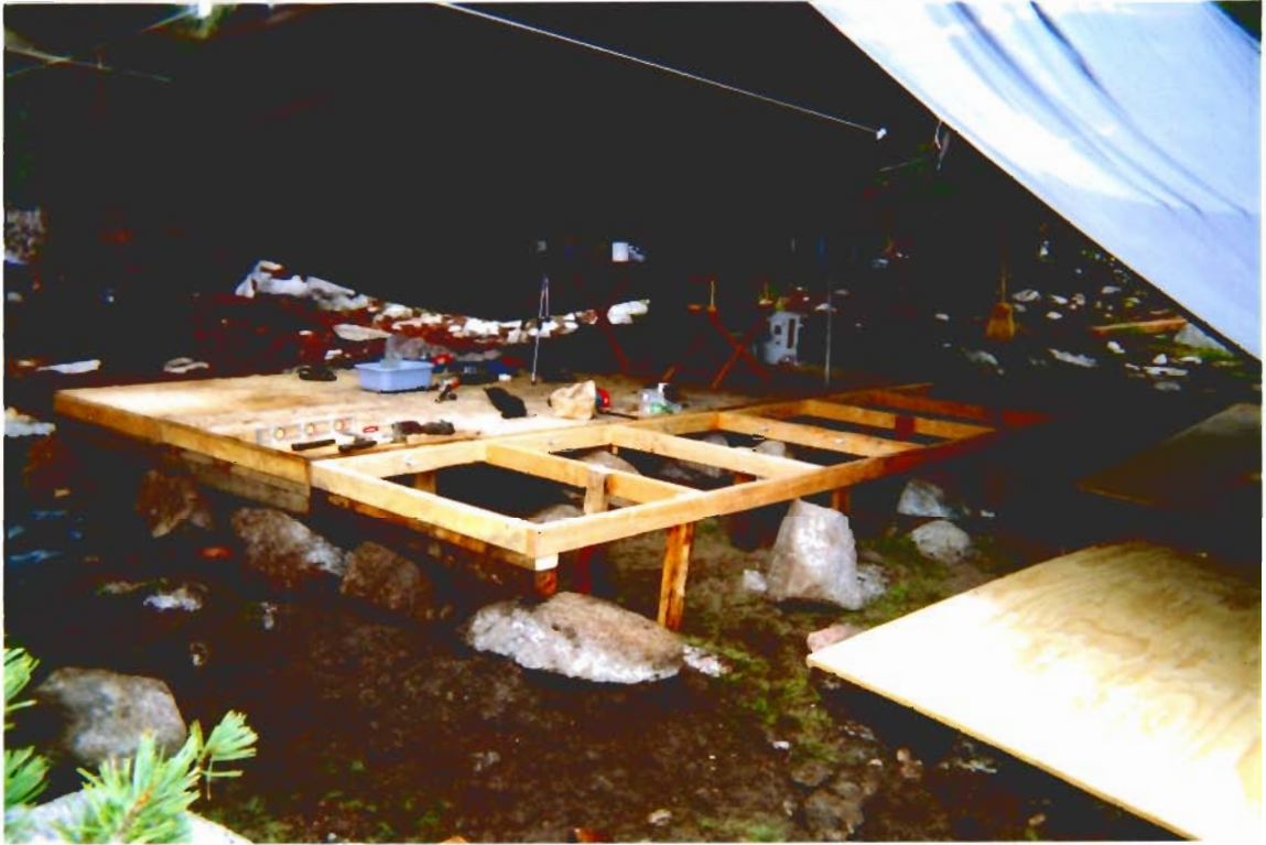
Frame bolted together with support bracing
