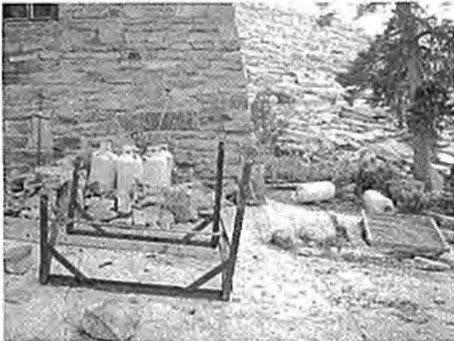
Partially removed frame
