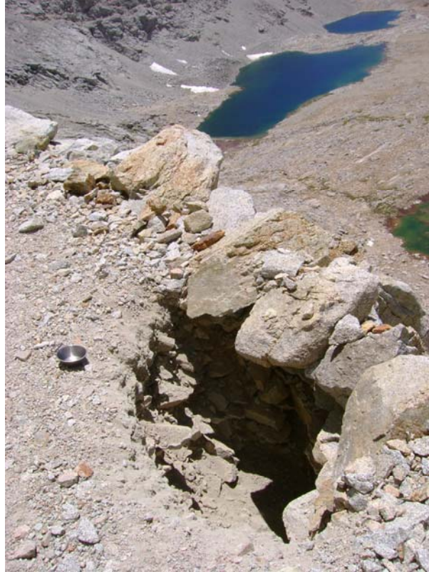
Cavity eroding the John Muir Trail south of Forester Pass
