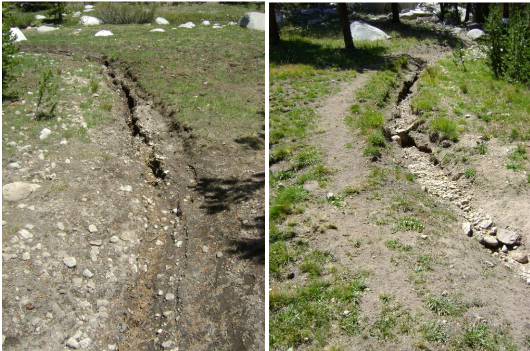
Army Creek Crossing in June (left) and August (right) with parallel trail and further erosion developing due to unrepaired water damage
