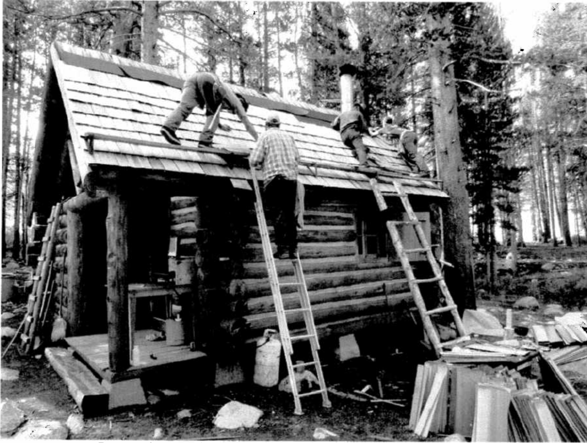
Construction crew installing new roof on the Rock Creek Ranger Station
