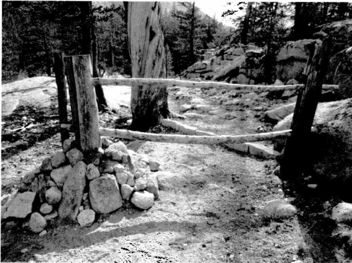
Rotted drift fence post repaired with rock pile
